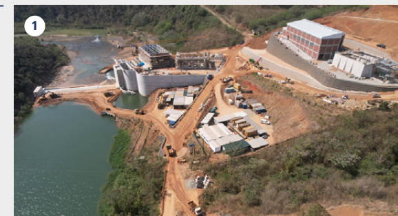
1 Integrated water infrastructure construction within a sensitive river environment.
