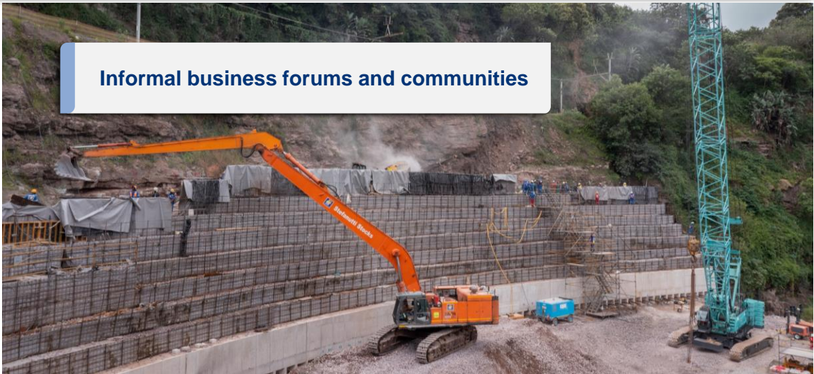
Slope stabilisation, Mount Vernon, KwaZulu-Natal
