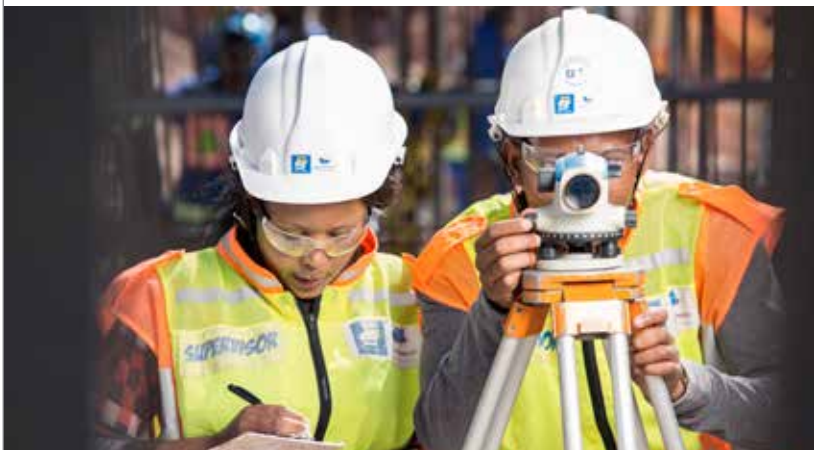
Junior site administrator Sherly Selahle and site engineer Stanley Tjabadi survey the concrete elevations of the foundation at the Medupi Raw Water Pump Station construction site.
