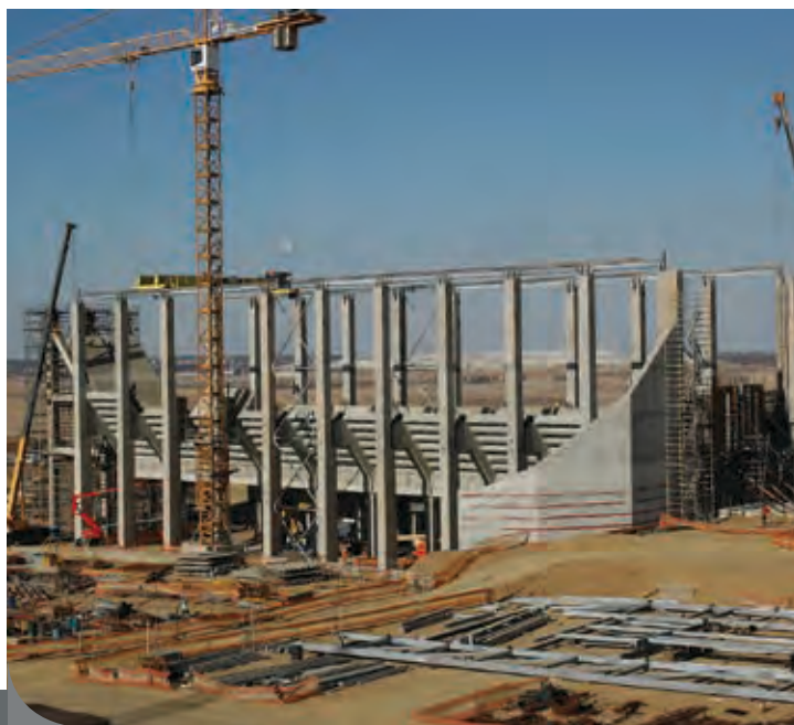
The Shondoni coalbunker under construction. Ikhaya Reinforcing is supplying the rebar for the project.
