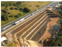
N2 ROAD EMBANKMENT
