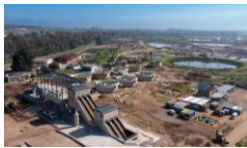
PAARL WASTEWATER TREATMENT WORKS
