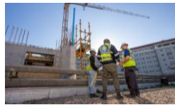
ALTERATIONS TO GROOTE SCHUUR HOSPITAL
