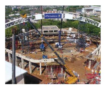
The complexity of casting several structural steel elements into the buttress columns (each weighing 4.6 ton), through a network of reinforcing bars, coupled with the 3-5mm tolerance for HD bolts, results in a structure that is demanding to construct and requires acute attention to detail and surveying.
