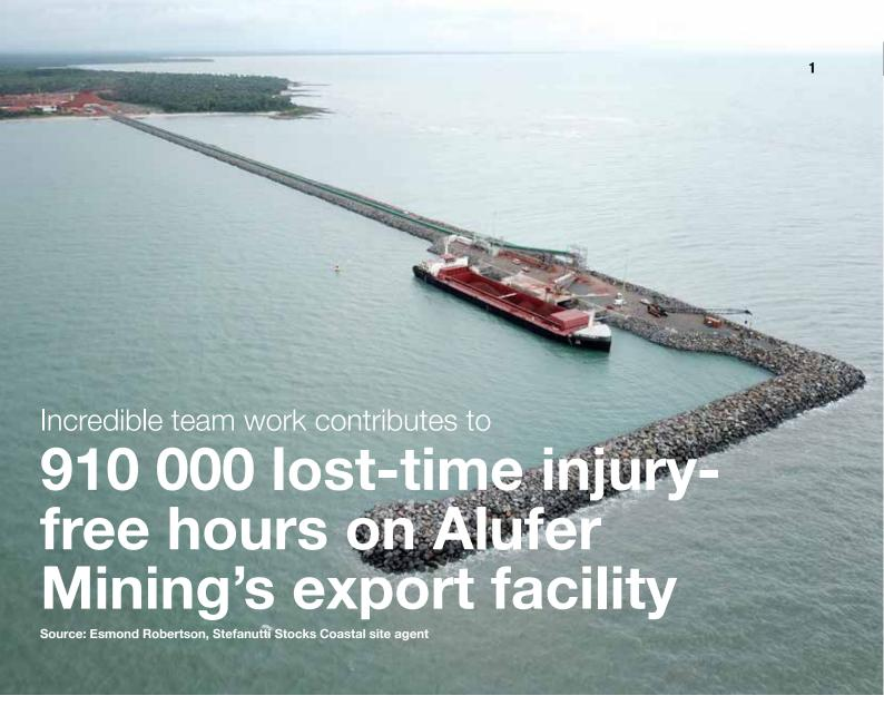
After working in a remote location in the Republic of Guinea for just under eighteen months, Stefanutti Stocks Coastal completed the construction of an export facility for Alufer Mining. The facility was required to accommodate a conveyor line and a telestacker, that would load bauxite onto individual barges berthed along the quay wall.
