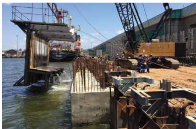
Stripping a cope shutter.
