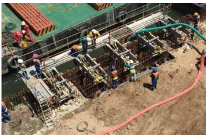
Dewatering and final preparations before a cope cast.
