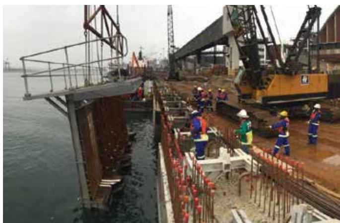
Fitting the shutter.
