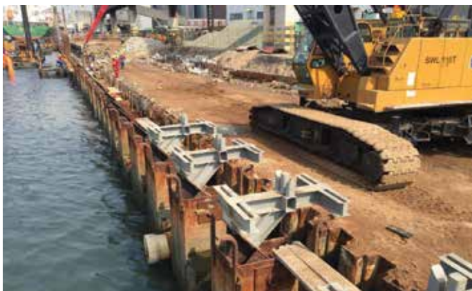
The pedestals in position and ready to support the shutter.
