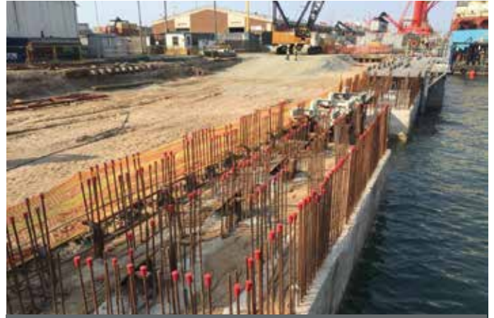
A completed cast with the shutter removed.
