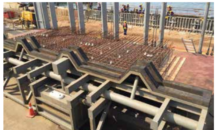
Rebar and foam seal prepared and ready for installation.
