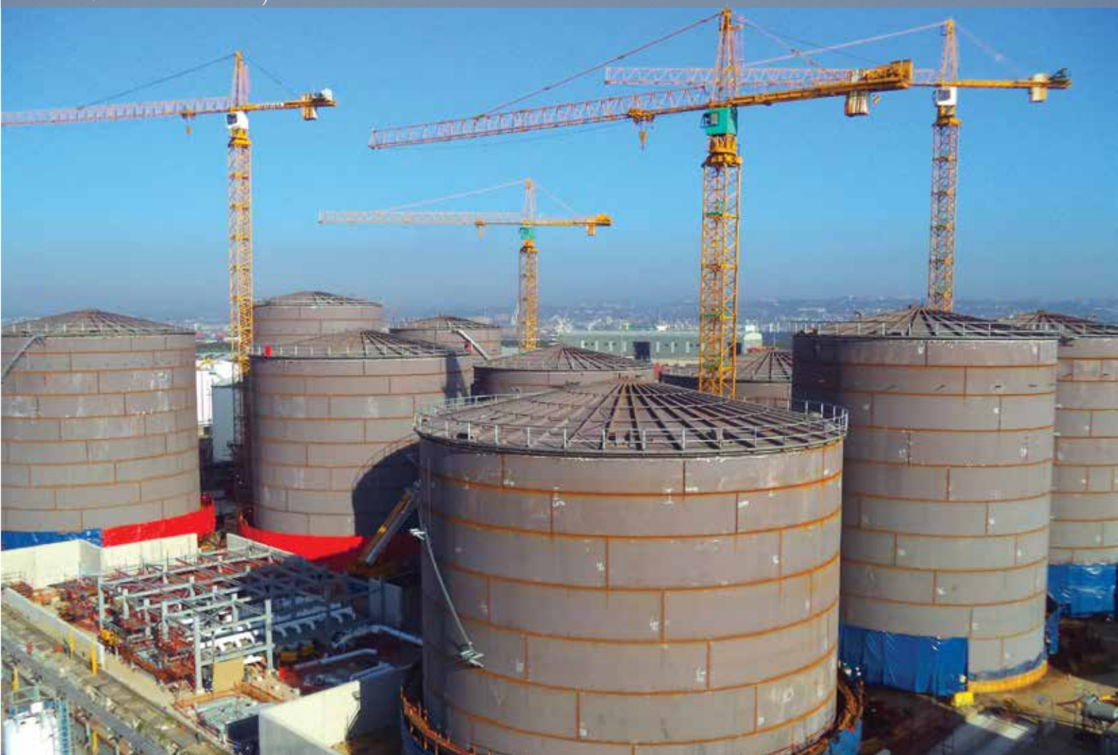
The Vopak Durban Terminal Growth 4 Farewell Tank Farm Project site, where Stefanutti Stocks Coastal is undertaking the construction of the tank bases, manifold, bund walls and ancillary works.
