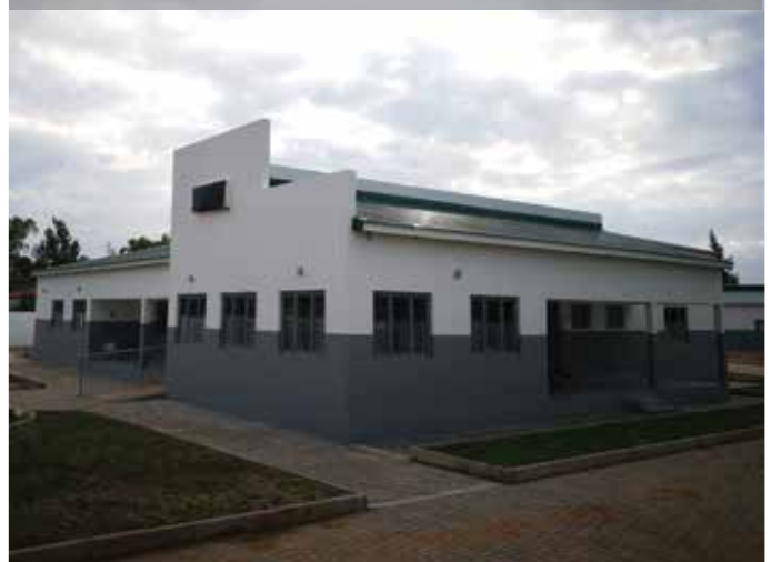
The completed Chiango Police Station.
